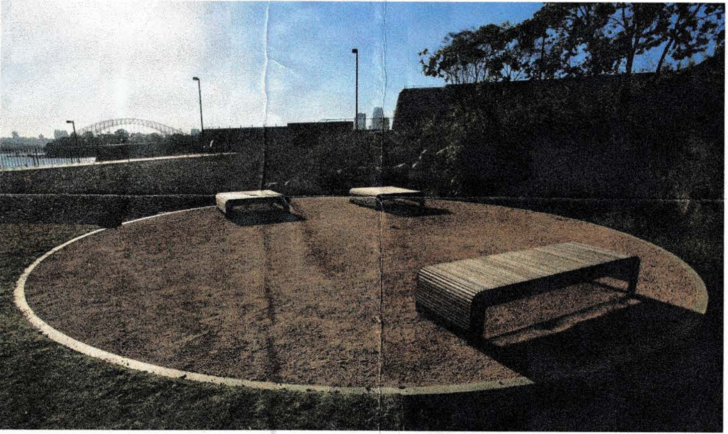
Seating and viewing area defined with decomposed granite and concrete circular edge
