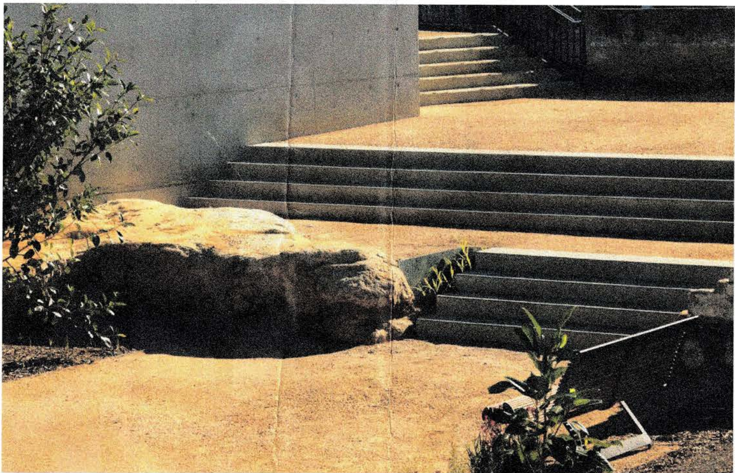
Stabilised decomposed granite surface in proximity to concrete steps and natural sandstone boulders
